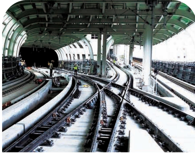
Double Slip Turnout 复式交分道岔
