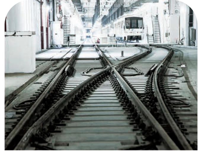
Double Slip Turnout 复式交分道岔
